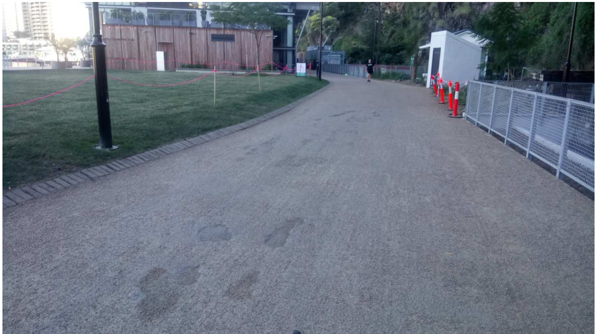
Figure 2 - Potholes in active transport corridor surface
