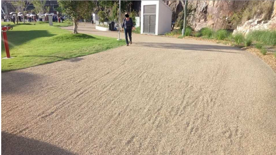
Figure 3 – Loose gravel surface of active transport corridor
