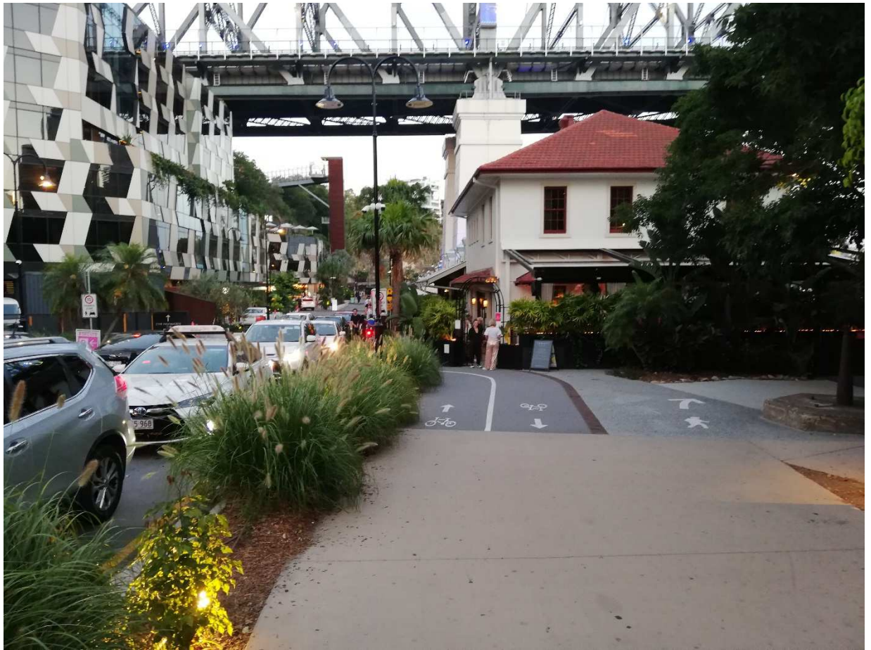
Figure 13: main pedestrian path blocked by restaurant, with many pedestrians choosing to mix with heavy traffic rather than take detour to the right
